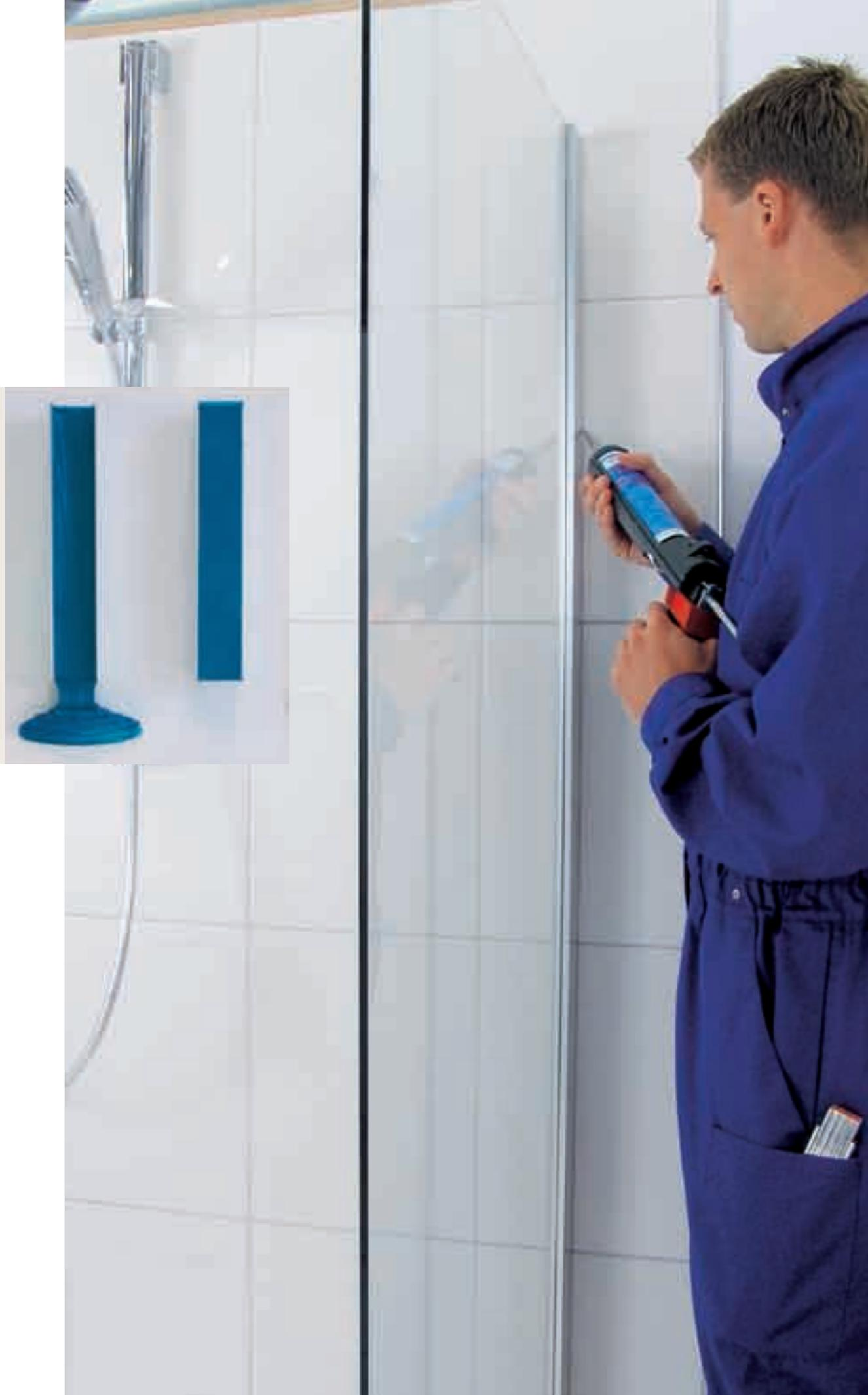
Processing of RTV one-component Silicone Sealants, e.g. for sealing showers
